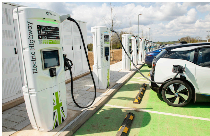
Rapid chargers like these new 350kW units at the Electric Highway charging hub on the M6 can recharge your electric car within minutes
